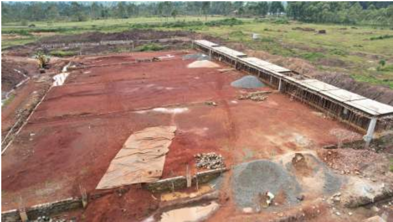
On-going construction of 8 units at Sironga industrial park
