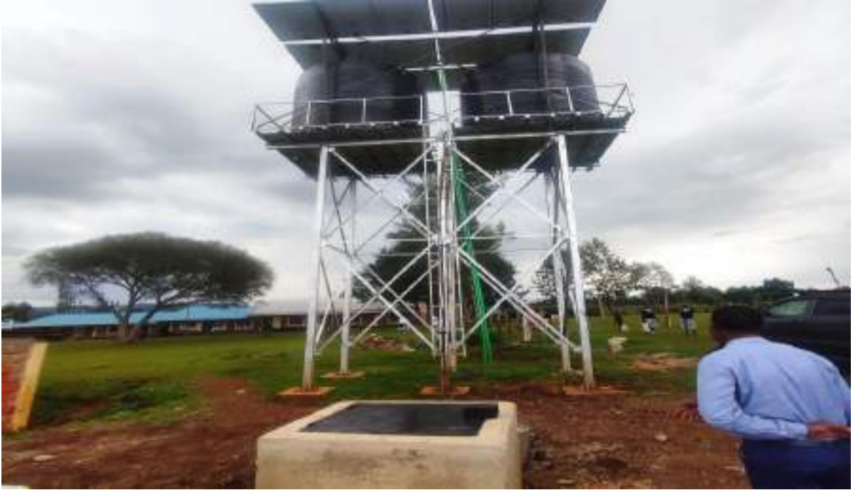
● Figure 5: Rionguti Borehole Magombo
