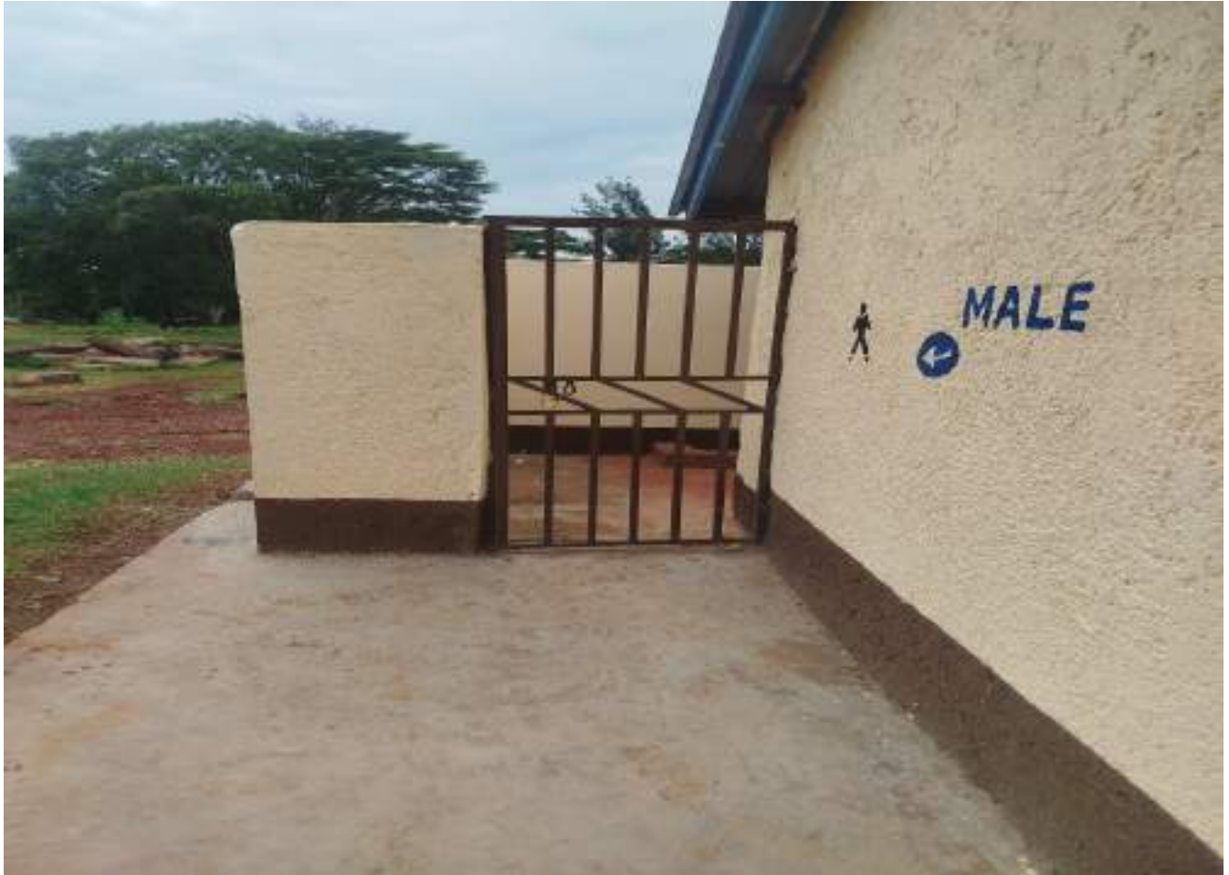
Renovation of Miruka livestock section pit latrine
