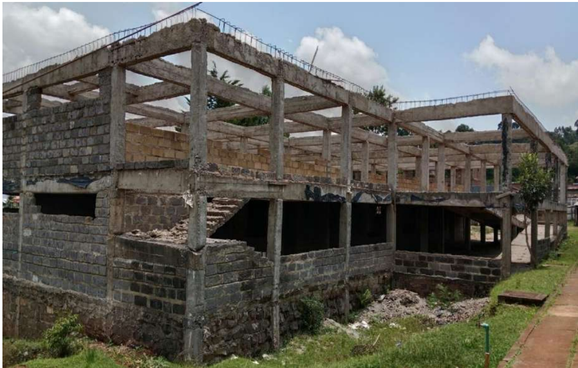
4. County Referral Hospital Covid-19 Isolation Complex
