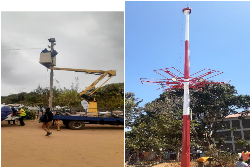
Repair and Installation of street lights and High mast lights
