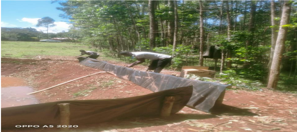
Picture 1.10: manga subcounty fisheries officers helping a farmer on dyke strengthening process.
