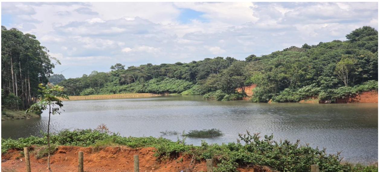
Dam/Water reservoir at Sondu, Climate change project
