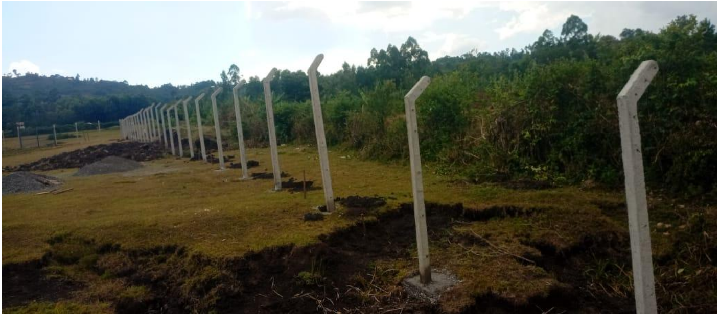
Ongoing restoration of Suguta valley in Magwagwa Ward
