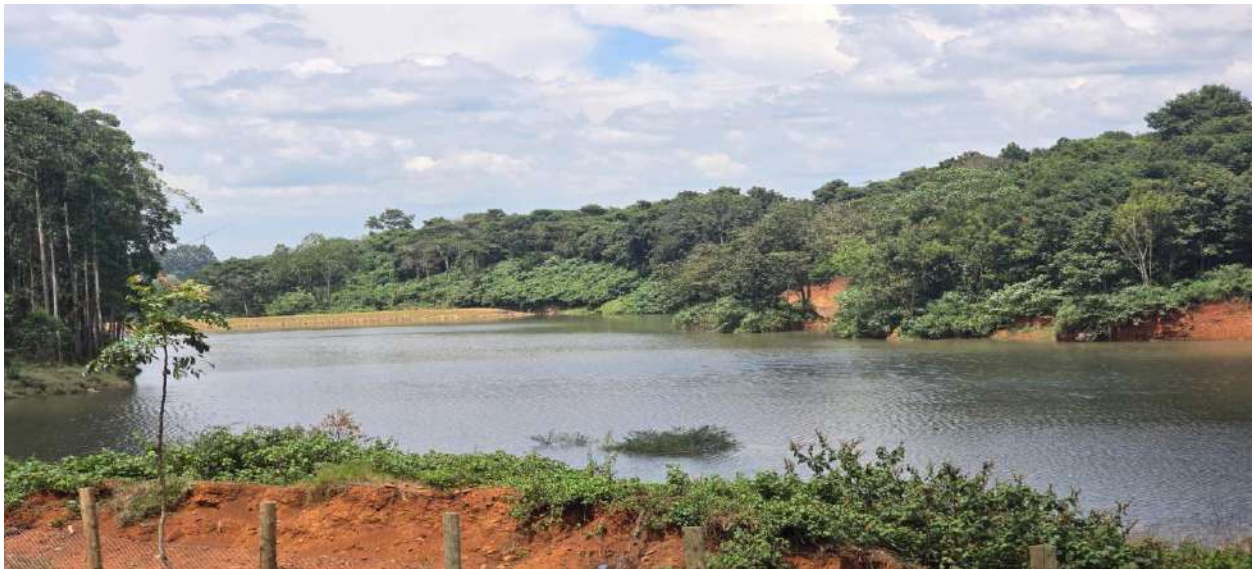
Dam/Water reservoir at Sondu, Climate change project
