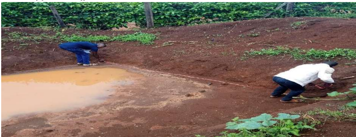
Picture 1.9: showing Nyamira South Subcounty Fisheries officer and his counterpart ward fisheries officer doing pond measurement to determine the size of the liner required to be fitted.
