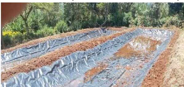
Picture 1.3 Kareha Investments Ltd's Matutu Farm two of the eleven [11] fish ponds fitted with pond liners and a water pan supervised by Borabu fisheries team.
